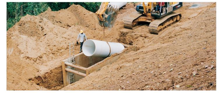
The first installation of Vylon Pipe occurred in 1987 for a direct bury gravity flow sewer. Since then, millions of feet have been successfully installed across the country. With its innovative I-beam construction and closed profile design, Vylon Pipe efficiently meets all the requirements published in ASTM F1803, including a minimum pipe stiffness of 46 psi.
